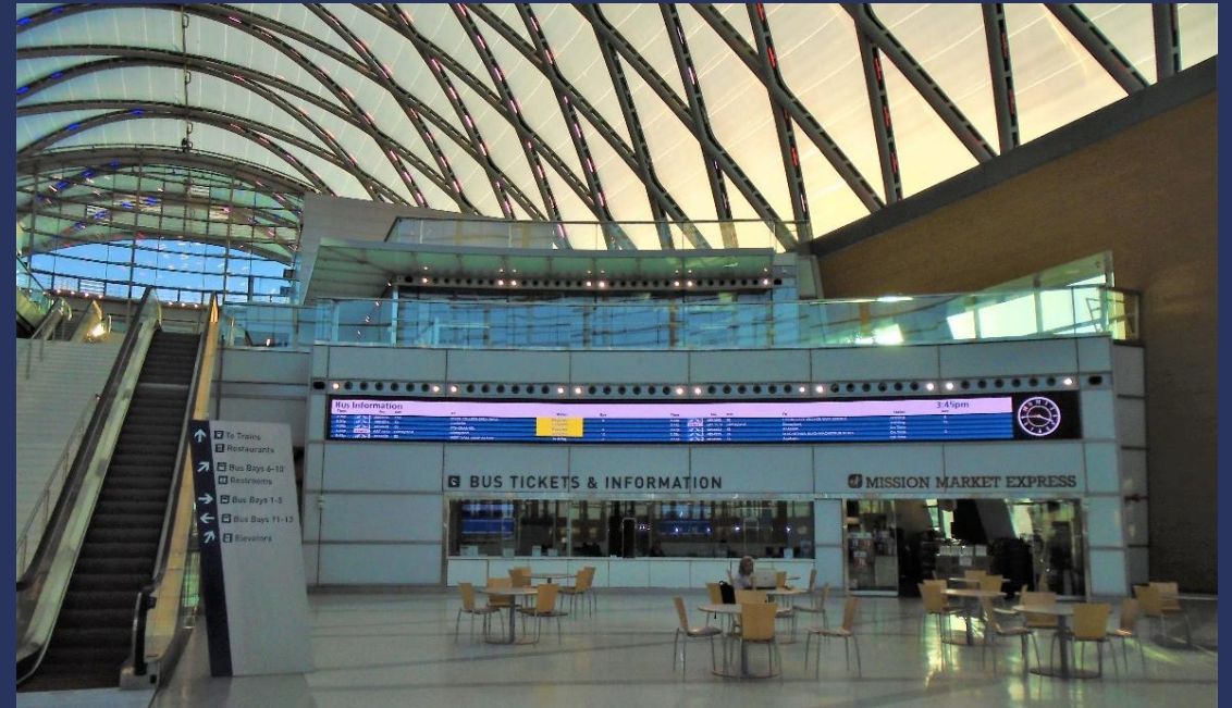
Anaheim Regional Transportation Intermodal Center (Credit: VHB)
