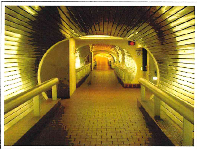
The pedestrian tunnel serving the train platforms at Union Station could be extended to the Long Wharf side of the tracks to improve access to Union Station from the South side of the City, and reduce traffic demand on Union Avenue.
